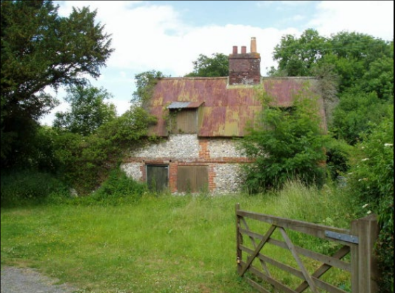
NO It's a listed building!
