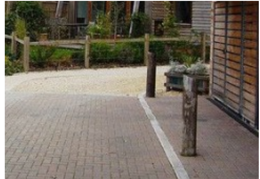
Reclaimed telegraph poles used as bollards at Great Bow Yard
