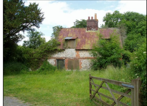
NO It's a listed building!
